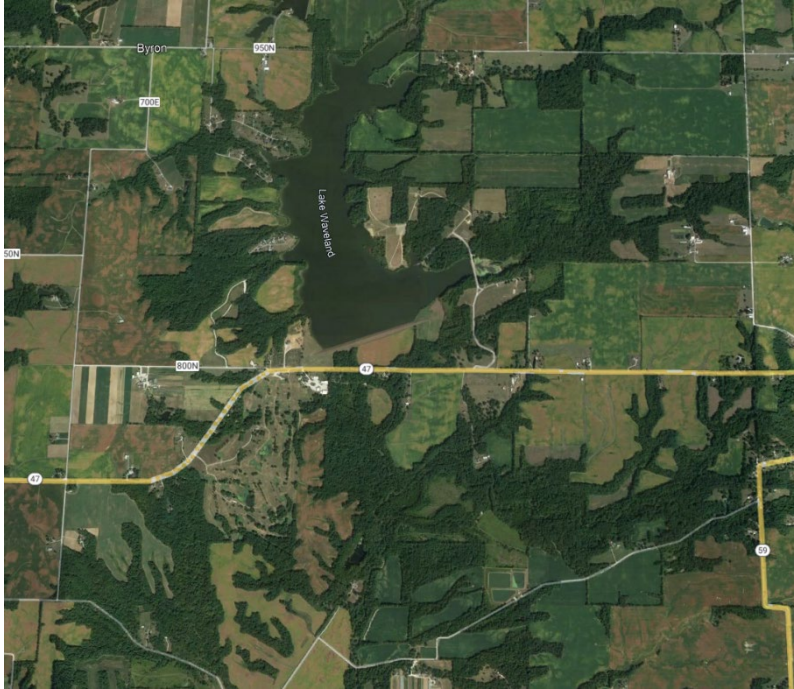
Figure 31 Waveland Lake and Dam
