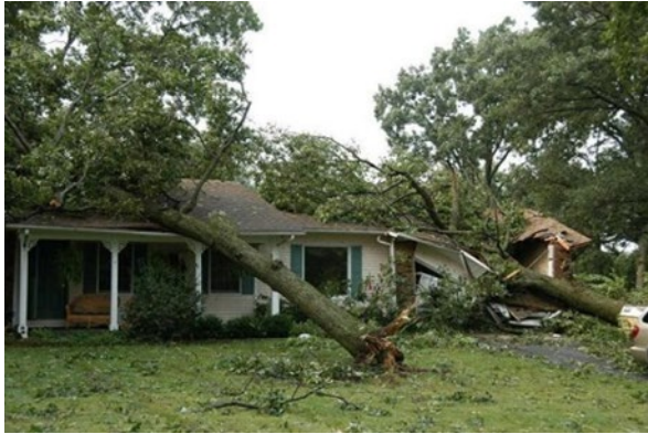
Figure 22 Home Damaged During Windstorm
