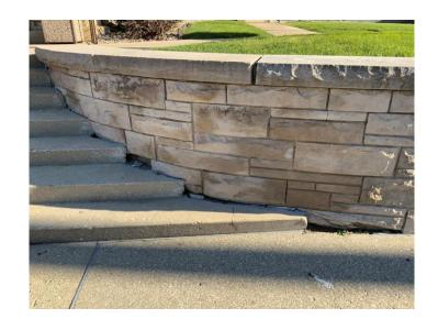
Low stone wall at west entrance needs tuckpointing and sealant at head joints some stone pieces have deteriorated and should be replaced
