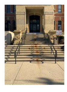
West entrance concrete stair is stained from where previous handrails were removed
