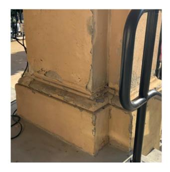
Skim layer over stone is failing and needs replaced
